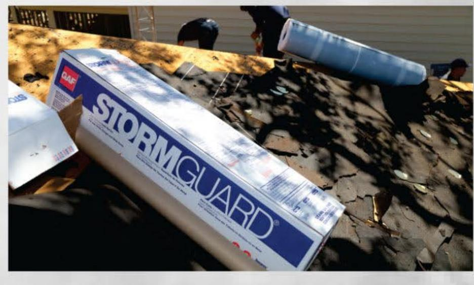
✓ Wall to roof and Chimney Flashings should be evaluated on an individual basis and replaced with either .032 Aluminum or 16 oz. Copper. Siding, Stucco and Brick conditions can severely impact the cost. Otherwise, these flashings will be painted, counter-flashed with StormGuard® or WeatherBlocker® and sealed with roofing cement.
