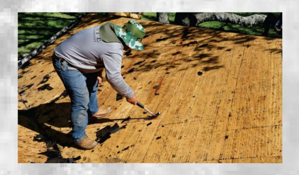
✓ Remove shingles and underlayment to expose deck – inspect deck for water damage or rotten decking. Replace decking as necessary.
