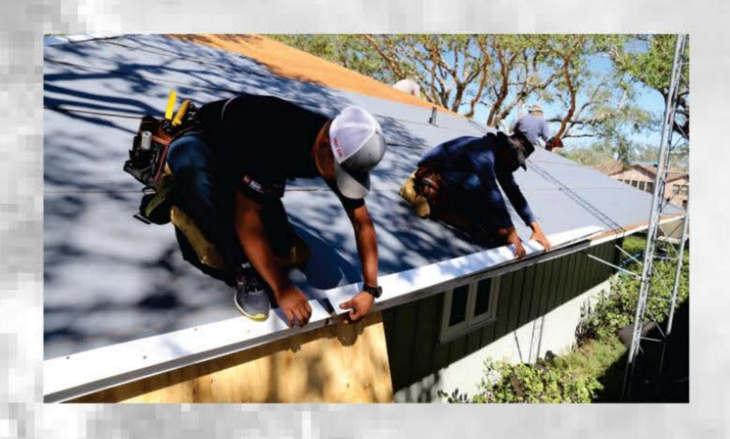
The DL Style Drip Edge will have a two (2") inch face. The drip edge will be nailed with a staggered nailing pattern – 6" on center.
