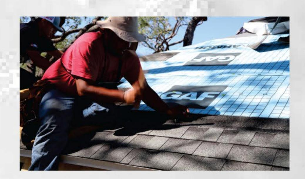
✓ Shingles (GAF Timberline HD Lifetime or Owens Corning TruDefinition® DURATION® Lifetime) are to be installed by hand nailing with six (6) nails per shingle. Nails are to be non-corrosive 1-1/4" Hotdipped Galvanized nails (or longer as necessary, to penetrate the roof deck). (Stainless Steel Nails are optional.)
