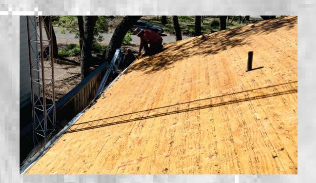
✓ Re-Nail decking with 2-½" Electro-Galvanized ring shank nails to meet current building code and Texas Department of Insurance Windstorm Certification requirements.
