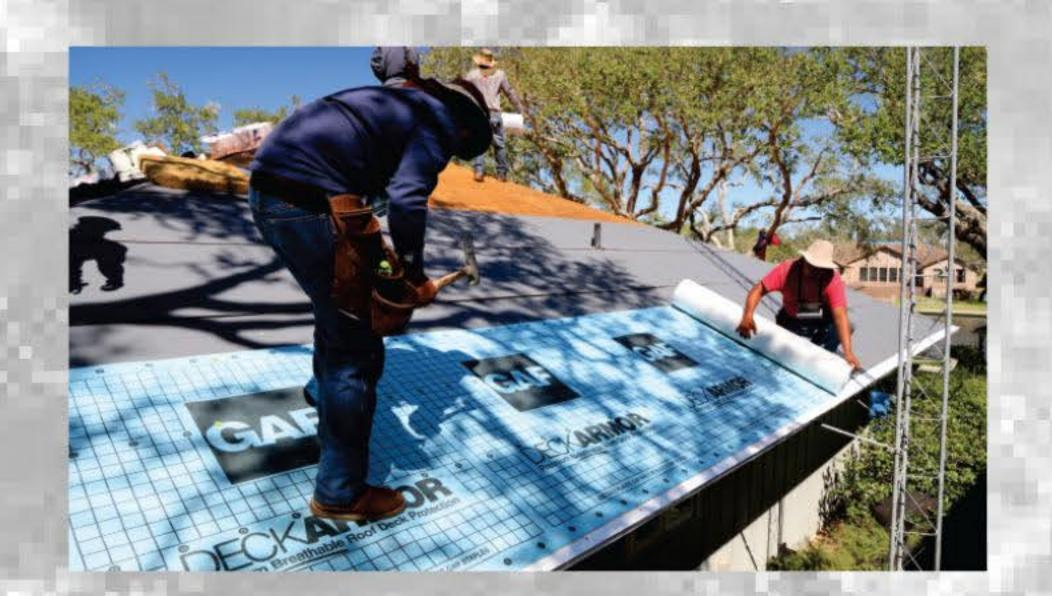
✓ Install synthetic underlayment over fully adhered underlayment over-lapping eave drip edge by two (2") inches and exposing lower row of nail heads. Install synthetic underlayment under the drip edge at any rake conditions.
