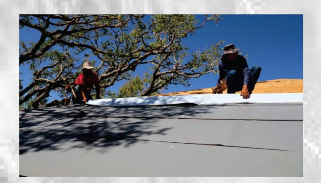
✓ Install fully-adhered 'Ice & Water Shield' product — GAF StormGuard® or OWENS CORNING WeatherBlocker®, installed under a four (4") inch (on decking) DL Style Drip Edge at both rakes and eaves.
