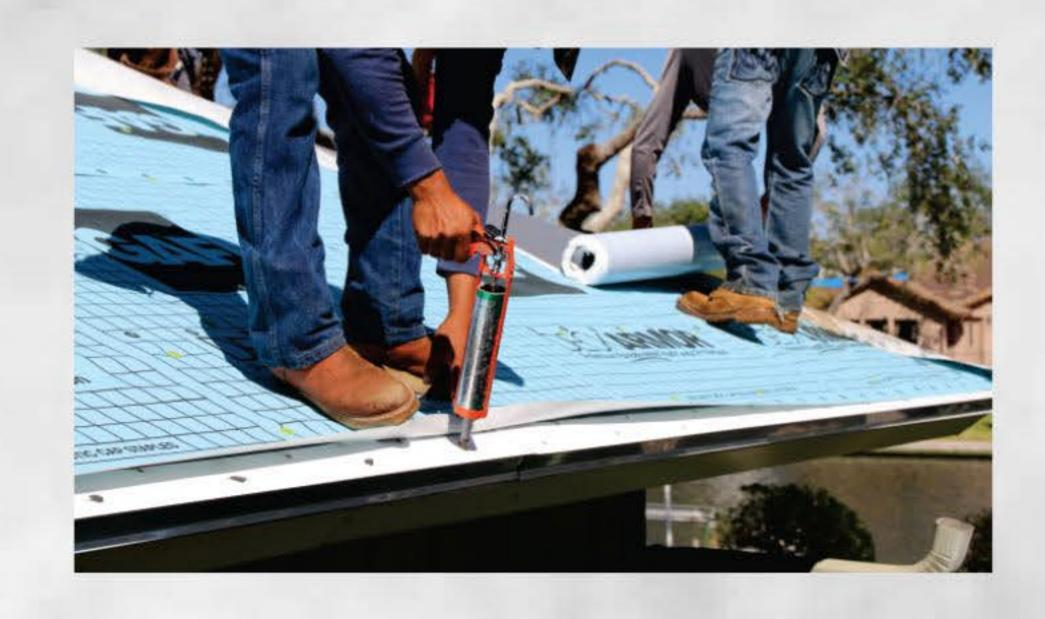
The nail heads closest to the edge will be hand sealed with a 'dob' of roofing sealant.
