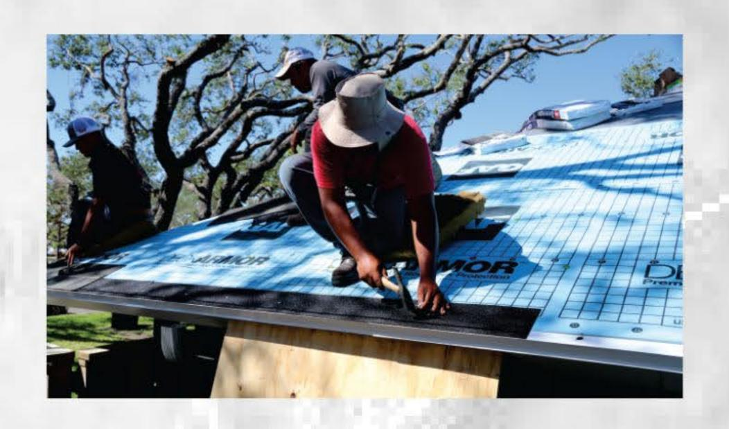
✓ Install (manufacturer's system matching) selfsealing Starter Strip to drip edge after a 'dob' of roofing cement has been applied to each nail head on the outside edge row of nails on the drip edge. Starter Strip is to be utilized at both rake and eave conditions.
